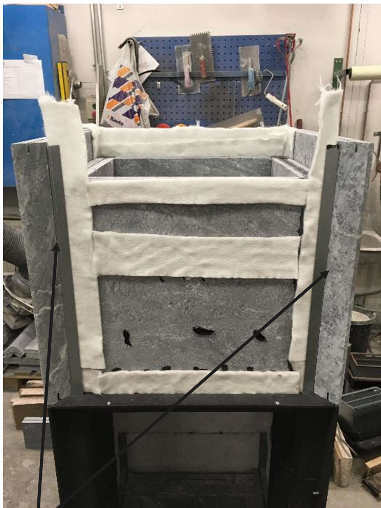
Put metal stripes (45 cm) to the miter corner
