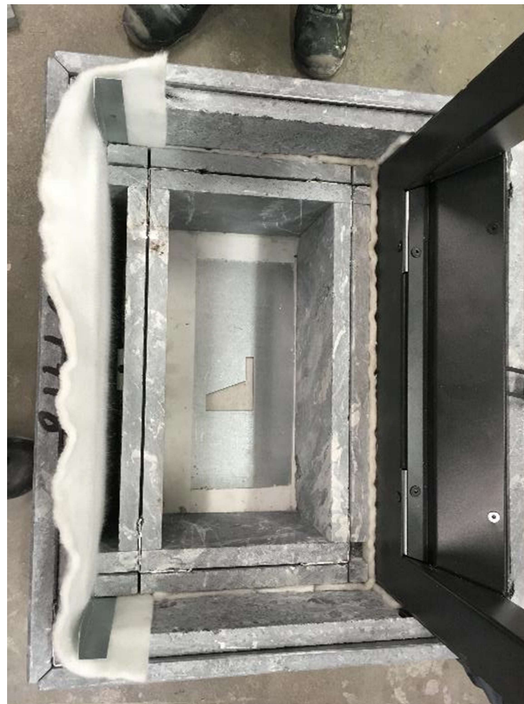
Insulate gaps besides the door unit
