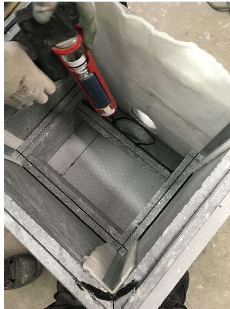
Tighten the air hole with silicone and inner corners
