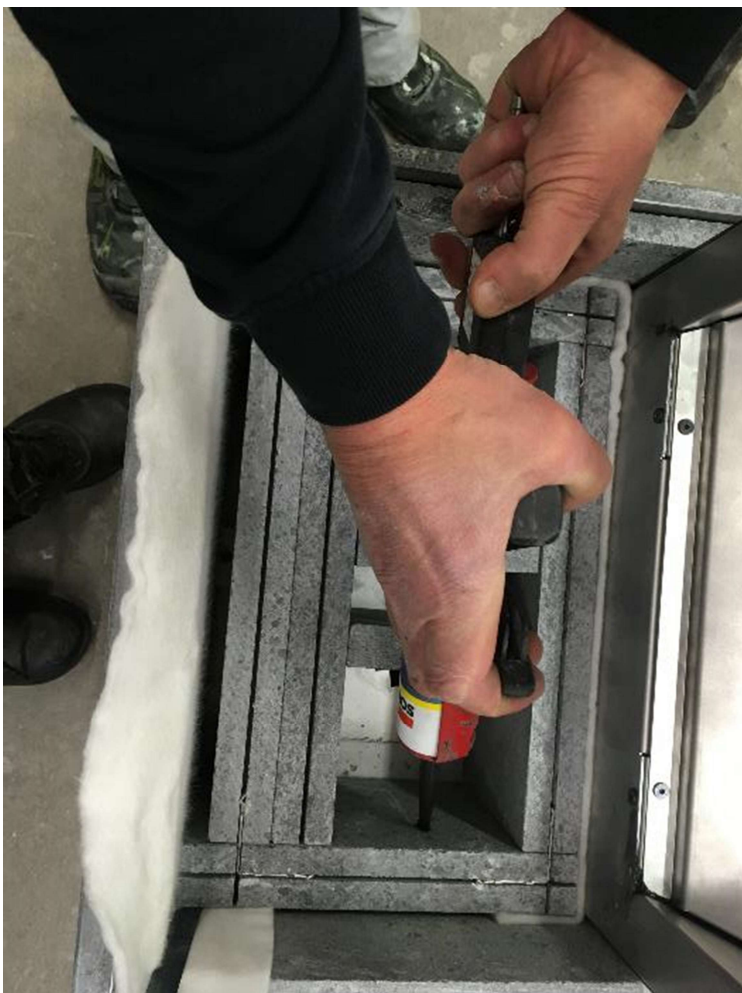
Use silicone taps for 30 mm stones
