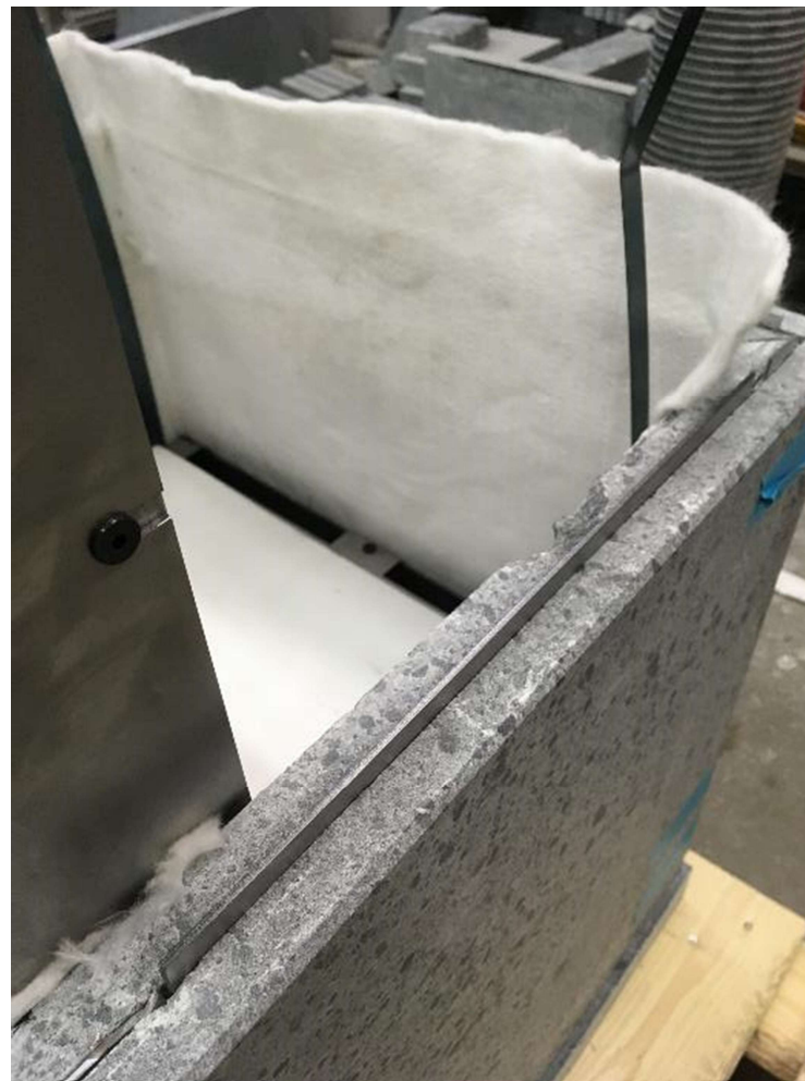
Install metals stripes to clip groove
