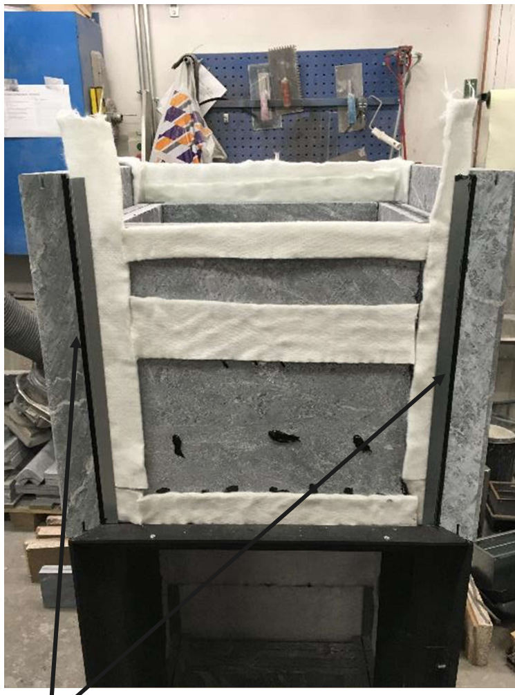
Put silico to the miter corner
