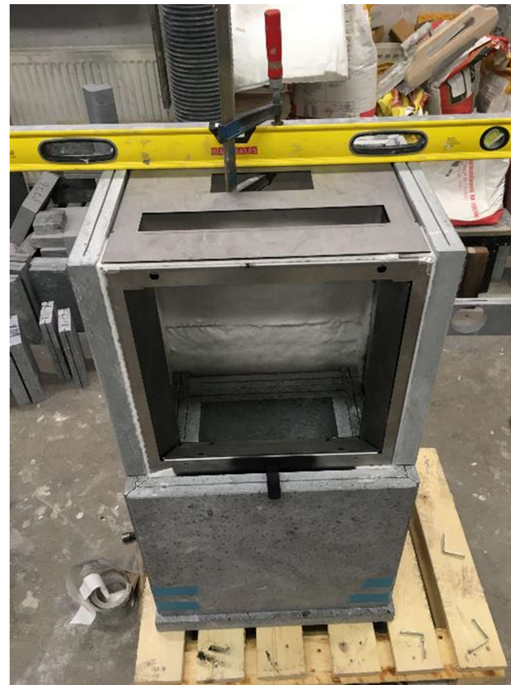
Install the inside stone plate, use tools to have it straight
