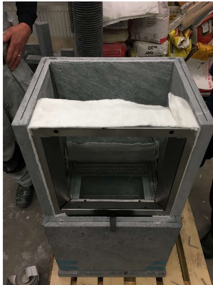
Use silicone for woools around door and install side stones
