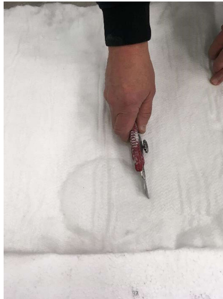
Cut the wool, in burning air from back side
