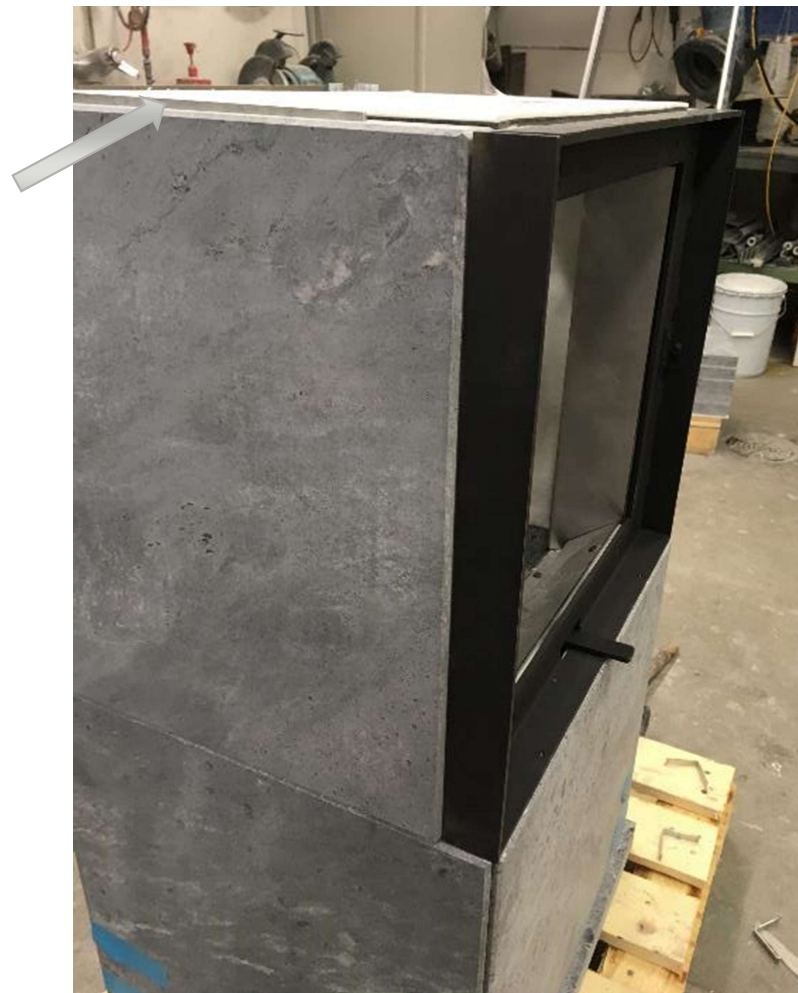
Remember install metal stripes to clip groove
