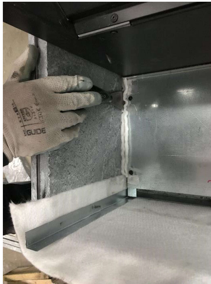
Drop door unit to the core
