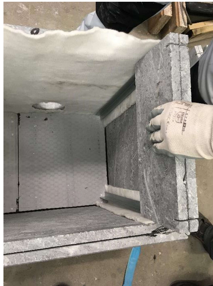
Put the side stone -> use metal stripes
